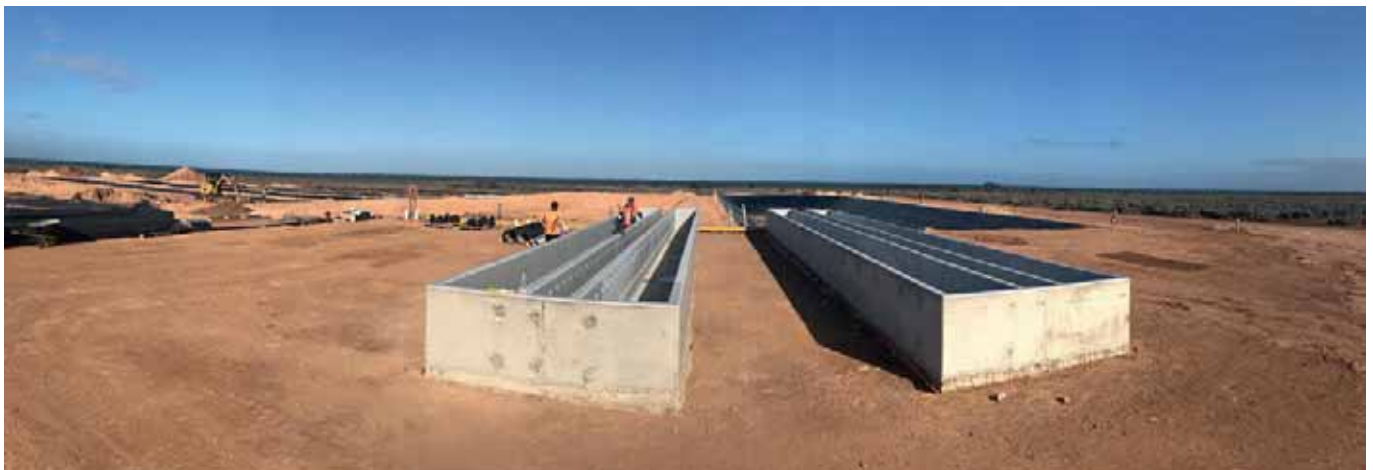
Raceways under construction at Eyre Shellfish in South Australia
